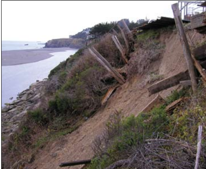
Coastal Commission approves replacement of failed retaining wall
